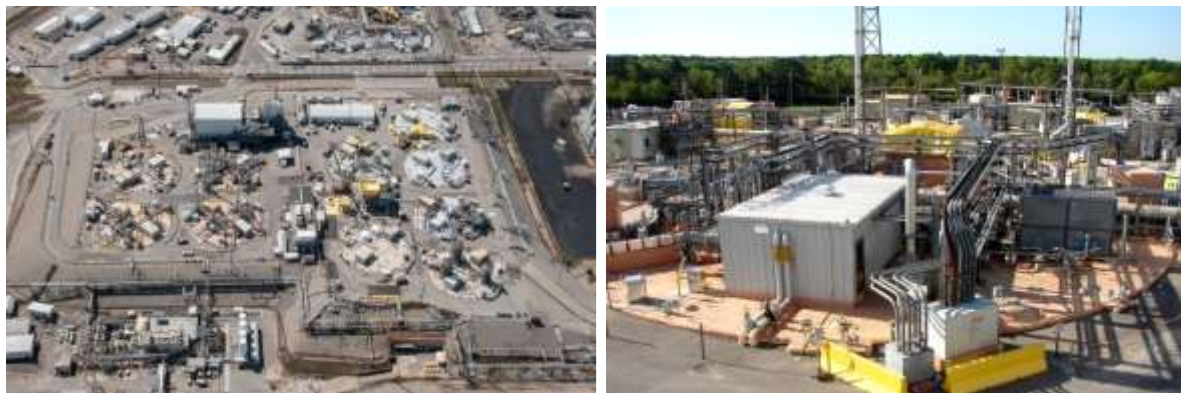
Figure 3. Tank 49H – Future Feed Tank for SWPF
