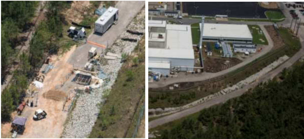
Figure 4. Installation of East Transfer Lines
