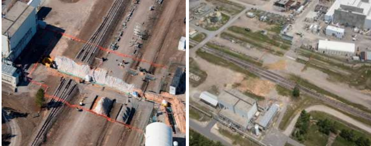
Figure 5. Installation of West Transfer Lines
